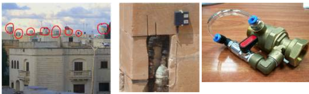
Figure 12: The pilot zone (left) where the UFR (right) was installed in Malta
